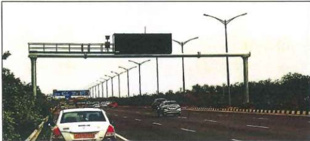
Figure 10:1 – Indicative Image of VMS Gantry
