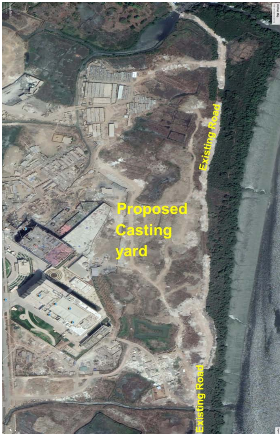
Fig 2.3 (b): Google image of Casting yard at Kavesar
