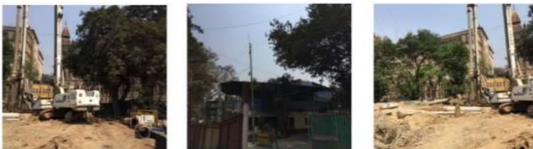
Figure 5.1 Site Photographs showing site conditions – CSMT Station
