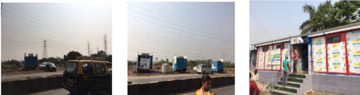
Figure 5.10 Site Photographs showing site conditions – Ganesh Nagar
