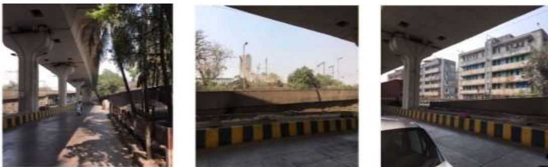
Figure 5.5 Site Photographs showing site conditions – Darukhana
