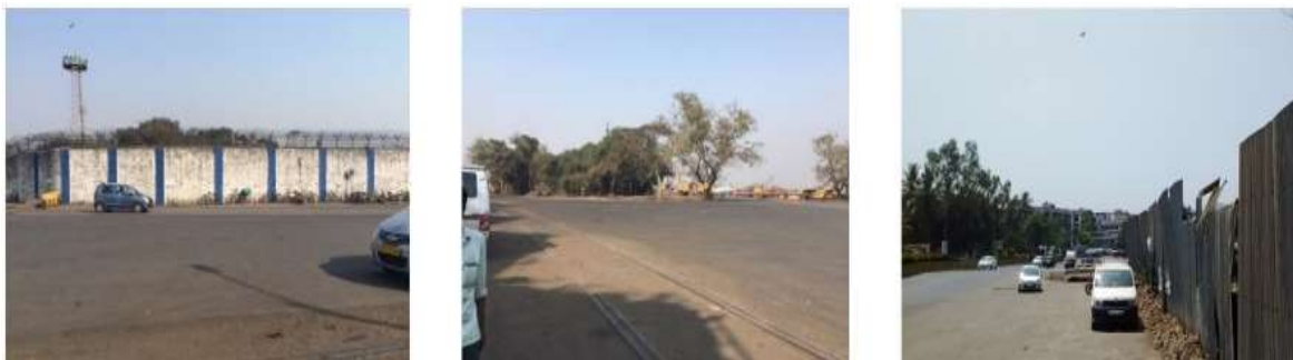
Figure 5.2 Site Photographs showing site conditions – Carnac Bunder
