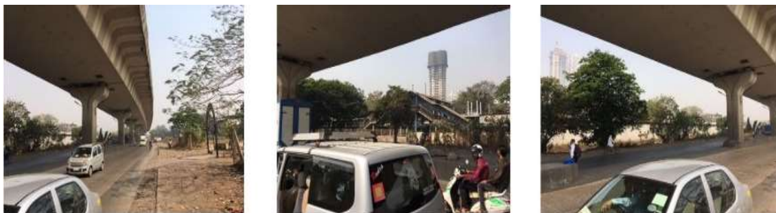
Figure 5.8 Site Photographs showing site conditions – Sewri
