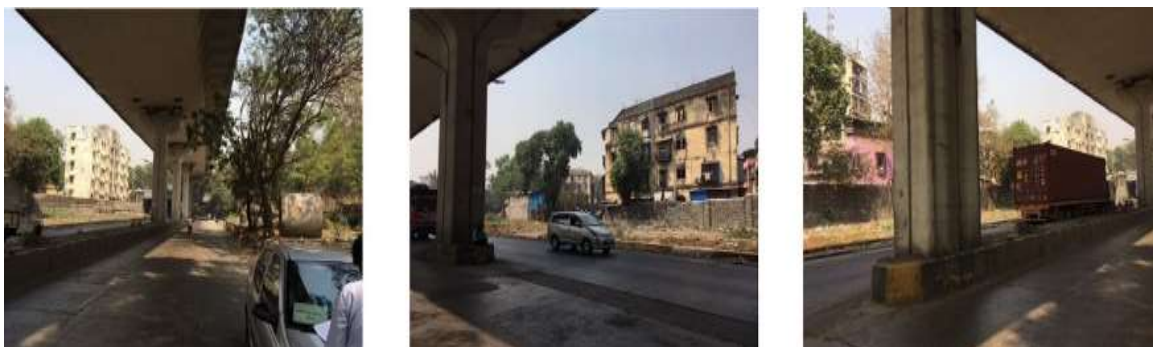
Figure 5.4 Site Photographs showing site conditions – Wadi Bunder
