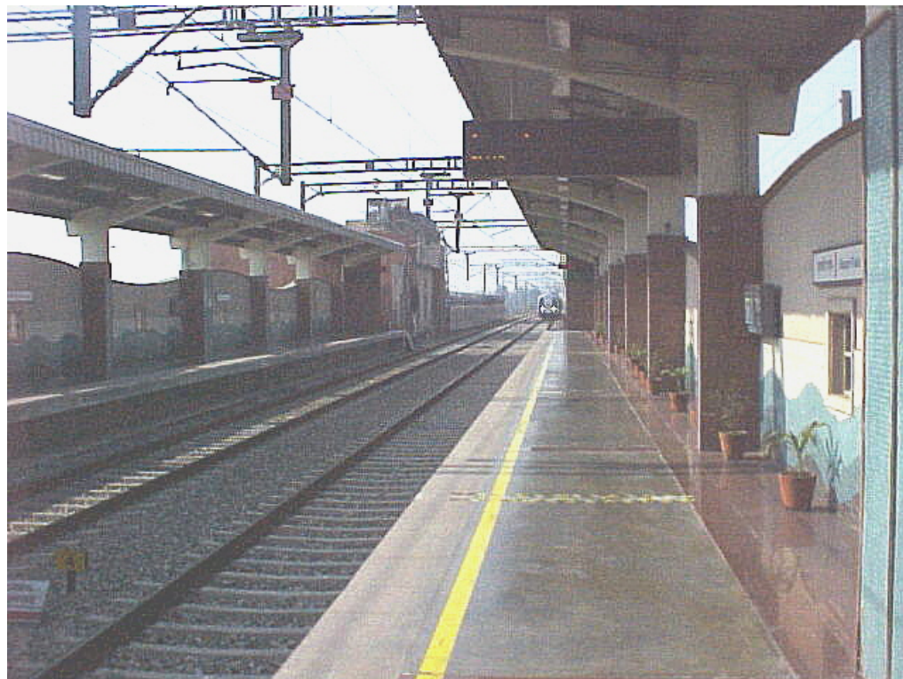
Typical 25kV AC Catenary Arrangement
